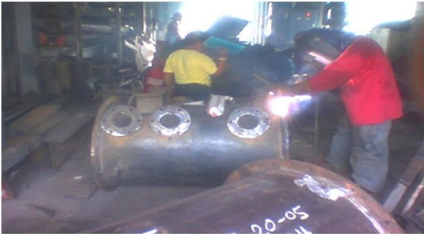
FABRICATION OF GASOLINE CYLINDRICAL TANKS
